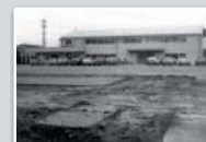
Construction of Hiroishi Plant
